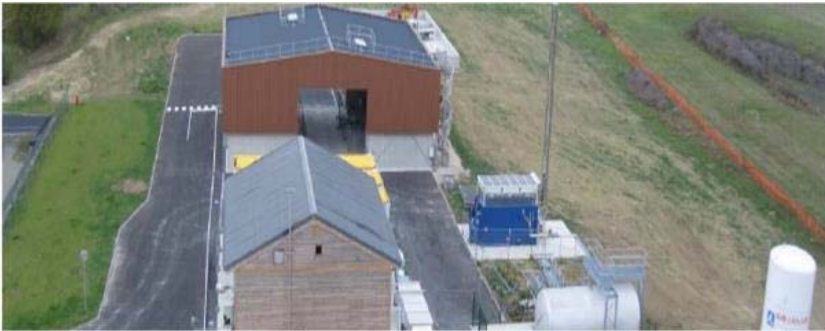
Figure 8: Industrial implementation at Oiry VERALLIA plant (France)
