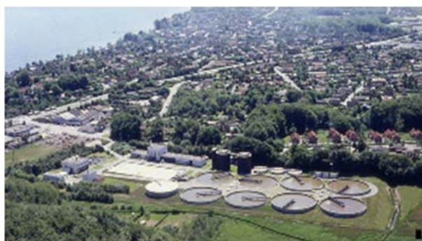
Figure 1: General view of Fredericia WWT- plant, including the upgrading plant at the bottom left corner. Source: Fredericia Rensningsanlæg.
